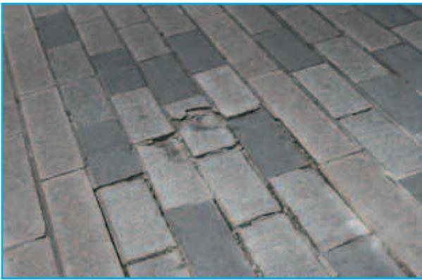
The photographs above show examples of how a scheme has failed as a result of poor design and construction. In the left hand case the restraining edge to the natural stone sets has failed under vehicle loading thus resulting in failure to the paved area. The right hand case is a further example of failure due to loading.
