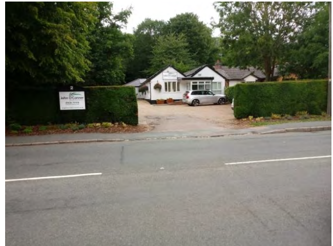
P6: HS16 Site Entrance from B197
