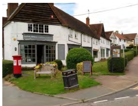
P20: Digswell - Woodside Road Shops
