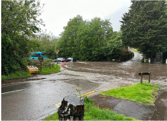
P3: Surface flooding – B197 at Oaklands
